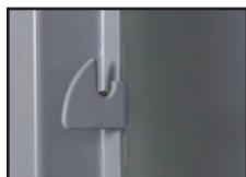
Main door latch hooks welded to frame
